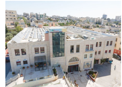
View of the LIFEGATE building from above
