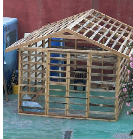
Another greenhouse is being built at LIFEGATE from old wooden pallets
