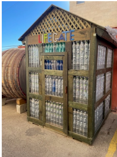
Building greenhouses from plastic bottles and wooden pallets "Lifegate environmental projects"
