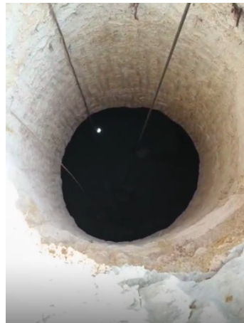
An underground water reservoir is chiseled out of the rock in Lifegate Garden
