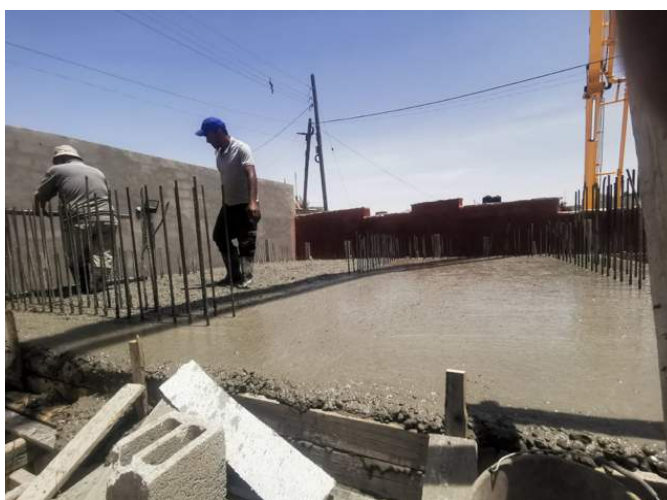
The ceiling of the shelter is concreted
