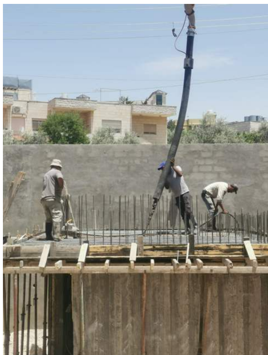
The ceiling of the shelter is concreted
