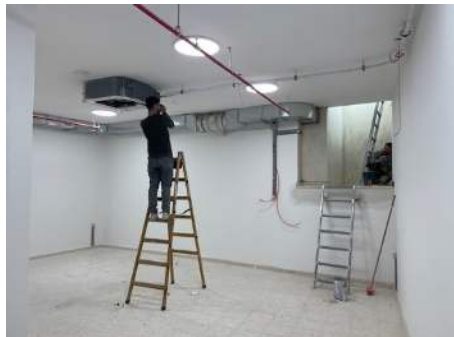
Air conditioning is installed in the shelters
